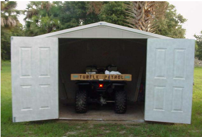
New storage building at Malacompra Fire Station
