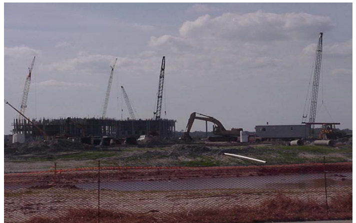
Harbour Village construction site
